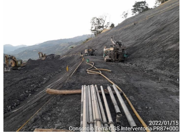
2022/01/15 Consortio Terra CGS Interventoria PR87+000
