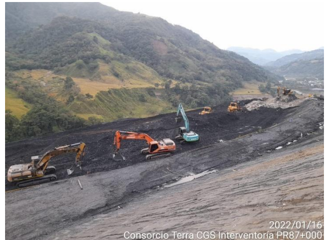
2022/01/16 Consorcio Terra CGS Interventoria PR87+000
