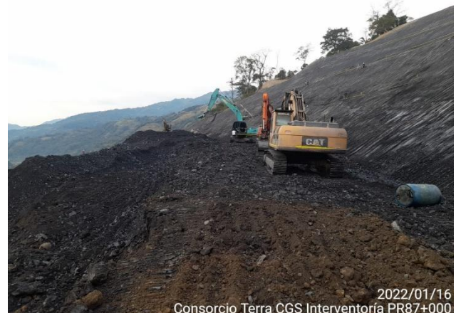
2022/01/16 Consorcio Terra CGS Interventoria PR87+000
