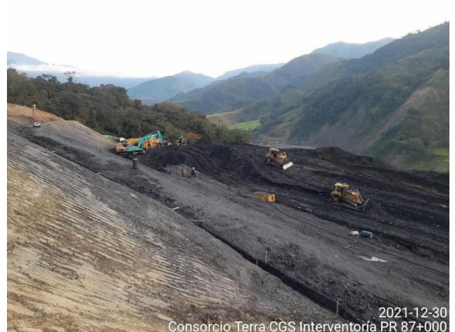
2021-12-30 Consortio Terra CGS Interventoria PR 87+000
