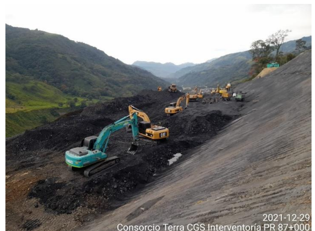
2021-12-29 Consortio Terra CGS Interventoria PR 87+000
